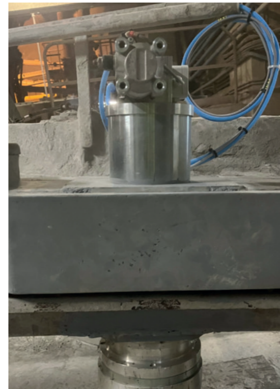
Installation on site
