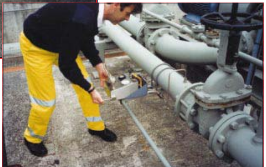
◀ Static Test Site Installation
