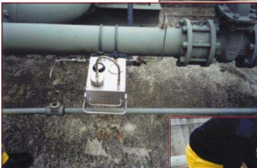
Permanently installed mounting tray and removeable Sampler ➤
