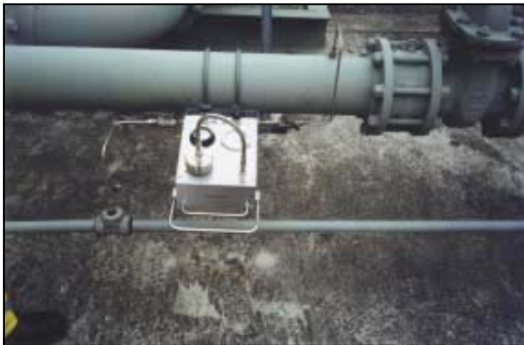
Static Test Site Installation
